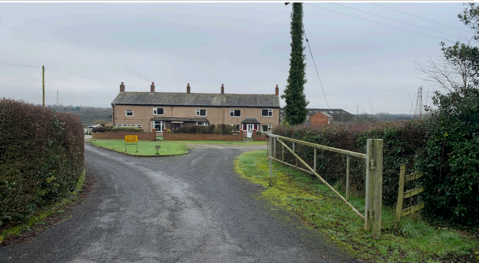
View from Hartshead Crescent looking at Existing Farm Structures
